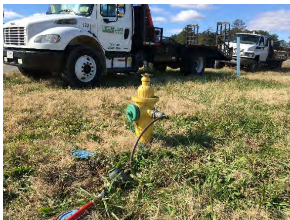
Hydrant Used for Dilution Water
