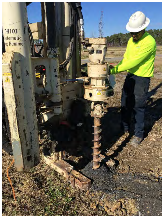
Deep Injection Point Drilling
