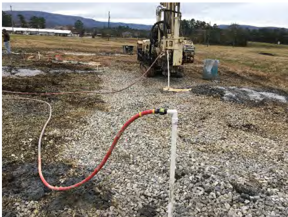
Injecting into Deep Injection Points
